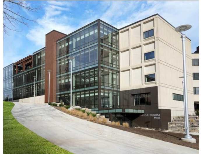
The newly renovated Dunbar Hall
